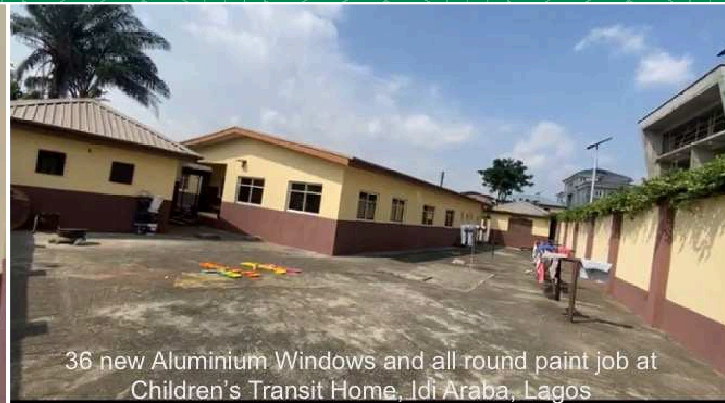
Renovation of Children's Transit Home, Idi Araba Lagos
